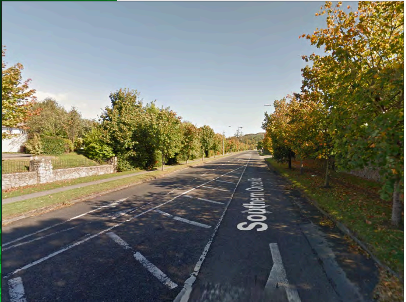
SOUTHERN CROSS ACCESS ROAD TO BRAY SOUTH
