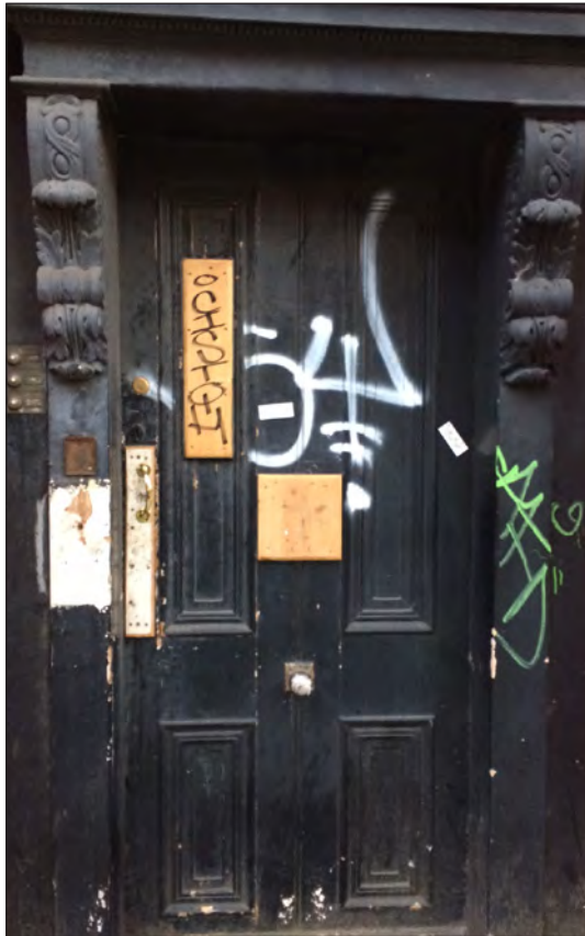
QUINSBORO RD SHOP FRONT - BEFORE
