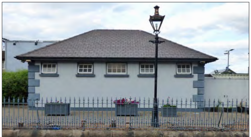
PLANTERS MADE FROM RECYCLED PALLETS / REINSTATED (LED) LIGHTS AT STATION
